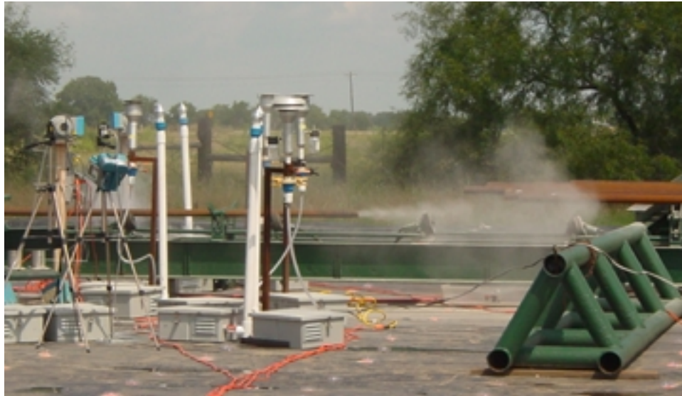
Figure 8. View of dust plume from oil pipe
